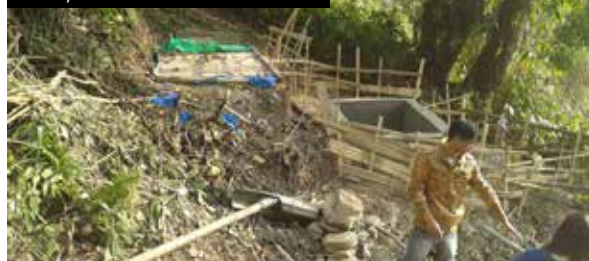
Newly constructed collection tank.
